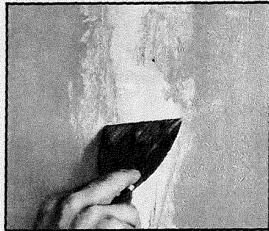
If shrinkage occurs, dampen patch area and fill cavity with fresh filler. Let dry. Sand smooth. Apply prime coat.
