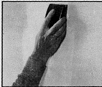
Use fine-grade sandpaper wrapped around a sanding block to smooth the patch and make it level.
