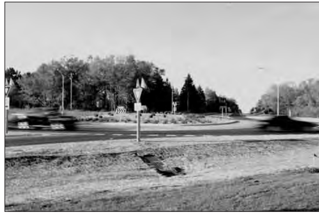
Kali photo/Nate Wisneski A roundabout was recently completed at the intersection of Highway 172 and County Road GE in Brown County.
