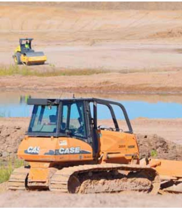
Kali photos/Travis Cottrell Full scale construction on the Oneida Lake has workers moving and compacting dirt in order to construct berms for tree walls and a fish spawning area. The ground is also being prepped for roadways, a beach, and boat launch. The Oneida Lake area is currently closed due to construction until further notice.
